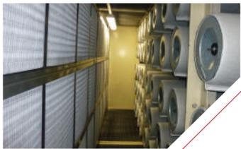
*A pre-filter removes hydrocarbons and oil particles from the air before they reach internal turbine components.*
